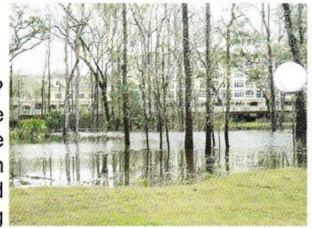
Retention pond overtopped the berm and flooded the lake in January 2006 after a 4-inch rainfall event. (Photo by Phyllis Saarinen)
